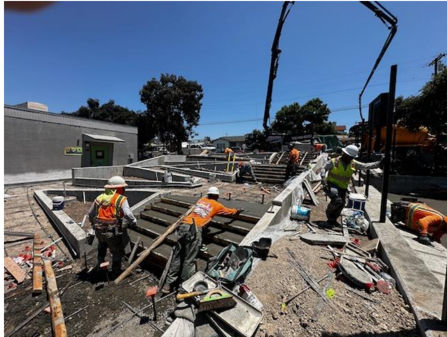
Security and Safety Entrance Improvements
