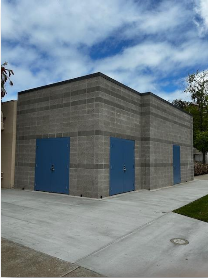
New Cooling Tower Enclosure
